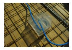
**4.** Connect the cable conduit. (Take care to avoid large gaps between back box and conduit)
